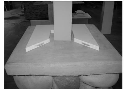
3) Slide ¾ cut base platform section around post.
