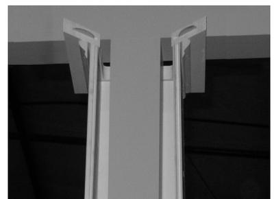
9) Slide ¾ cap platform section into place on top of column panels.\*
