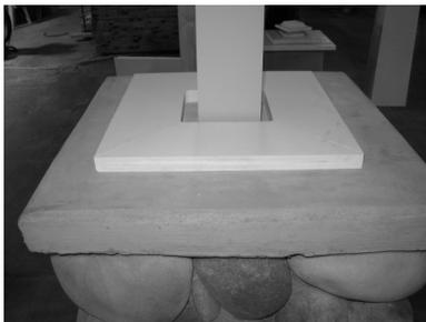
4) Glue base platform pieces using biscuits (supplied). Center and attach base to floor/pedestal with appropriate fasteners.
