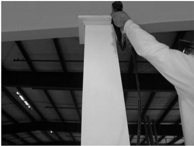
13) Apply glue to final 1/4 cap piece and biscuits and slide into place. Pin nail cap moldings to top of column.\*
