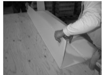
6) Assemble three panels, using E-Z Lock joints.
